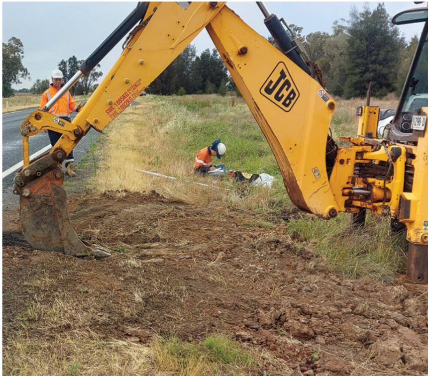
An excavator is used to dig a test pit so the existing road base can be examined
